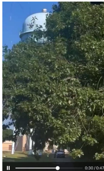
LEO Under Water Tower
